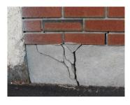
Foundations. When inspecting the exterior of your home, be sure to examine the foundation from top to bottom for masonry cracks. "Routine caulking by homeowners won't do the job," says Niles. "Hire a foundation specialist who can employ a two-part epoxy
